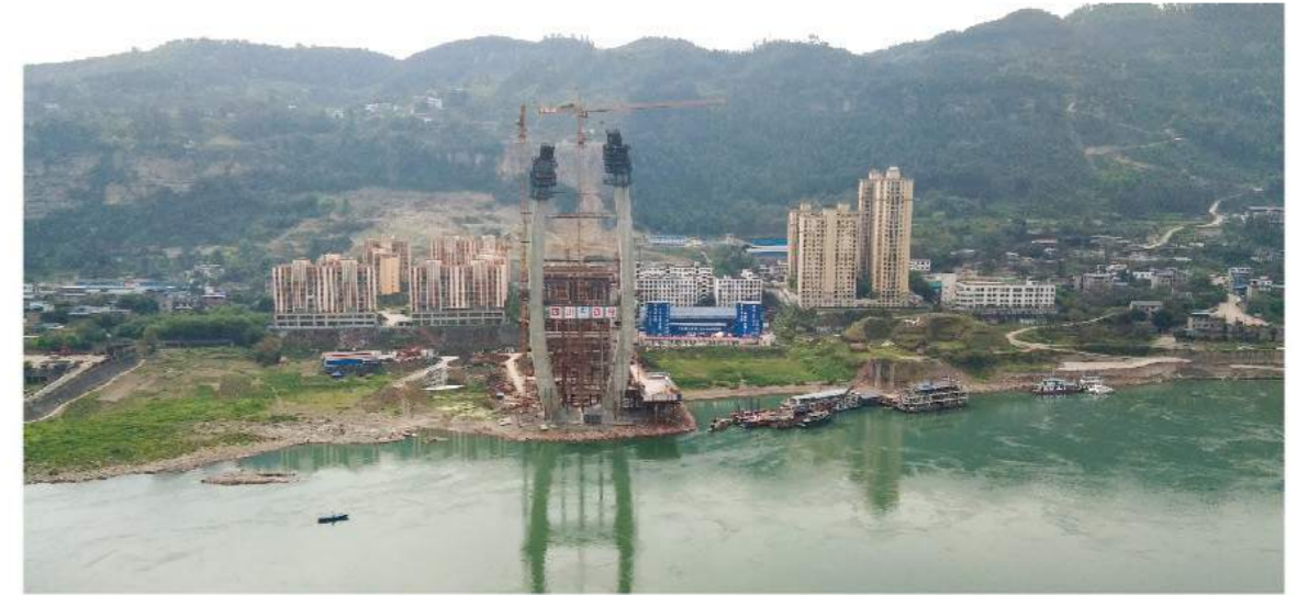
Project name: Yanpingba Yangtze River Bridge Contractor: Sichuan Highway Bridge Construction Group Co., Ltd. Products utilized: ACS, HCB-100 (Separate Truss Type)
