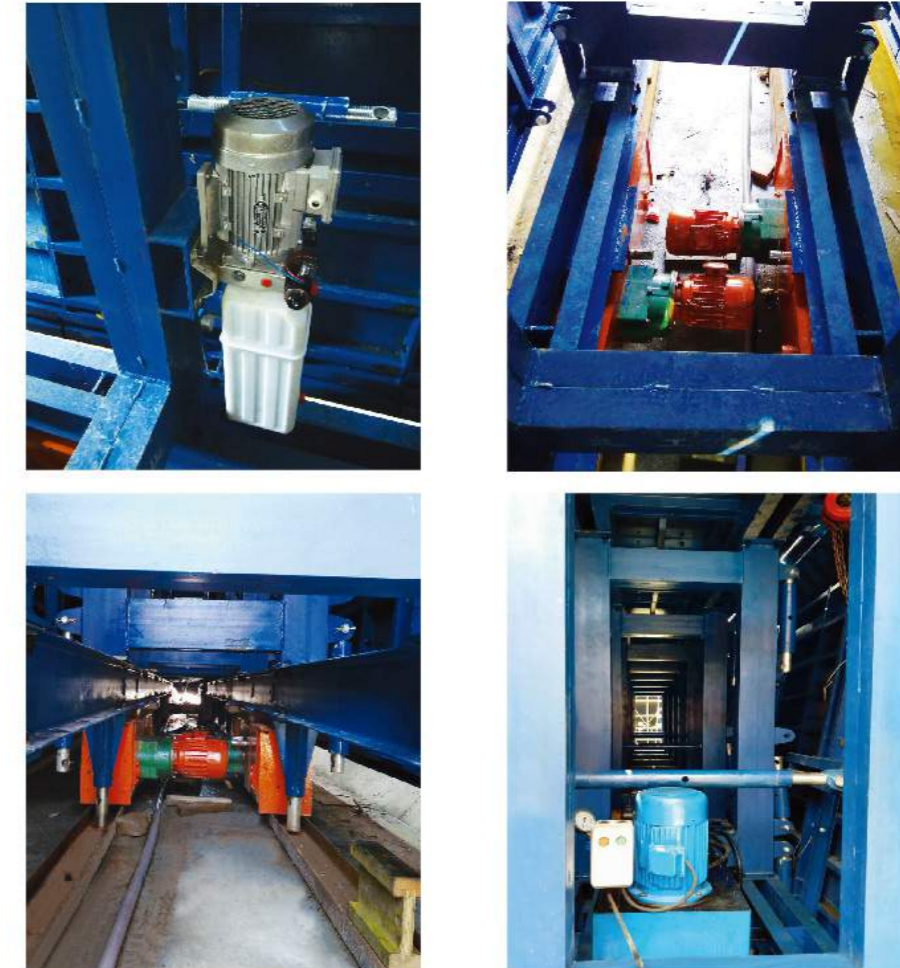
Installation of motor and circuit
