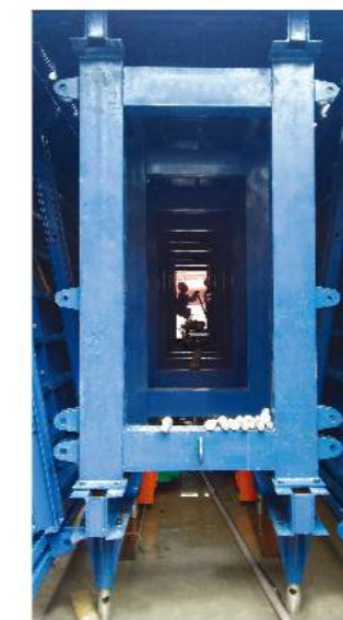
Connection of bottom stringer and gantry
