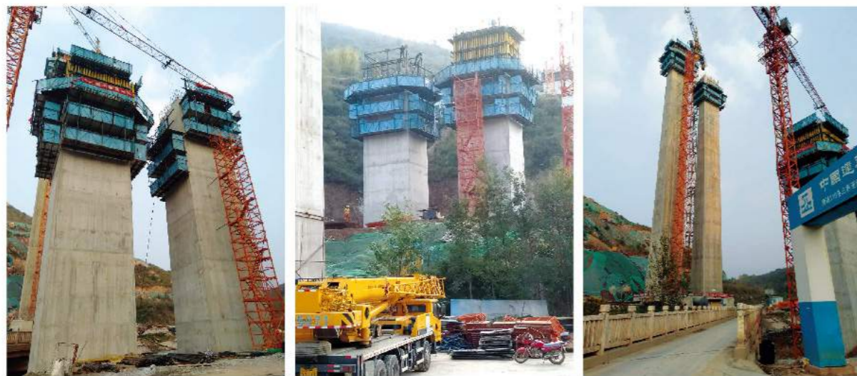
Project name: Shankou River Bridge Contractor: CSCEC Products utilized: CB-240(Diagonal Brace Type)
